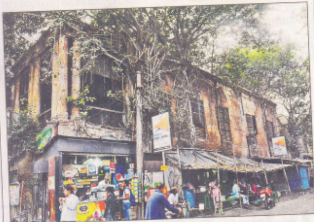
The dilapidated Registry Building. (Sudeshna Banerjee)
