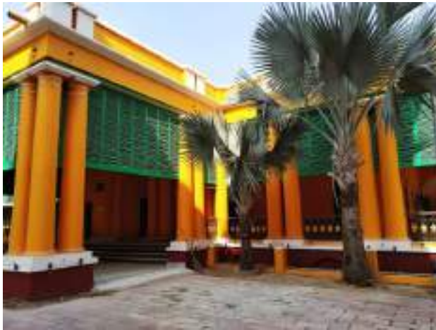
The heritage building
